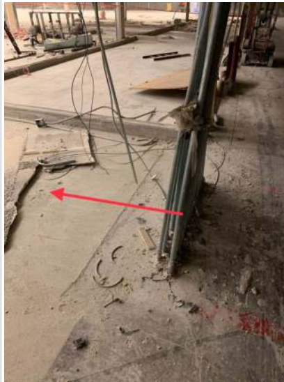
Underground conduits that avoid the trench path.
